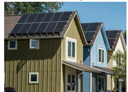
Residential PV System 14
