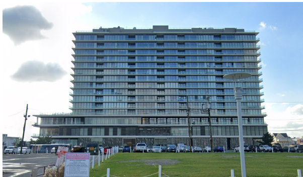
Figure 2: Asbury Ocean Club. Source: Google Street View.
