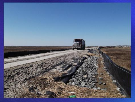
Avalon received permission to build a road to the Graven's Island CDF, located in Middle Township, owned by the Borough. Avalon exhaustively tested the materials at Graven's Island so they could be offloaded by a contractor. Approximately 70% of the 150,000 cubic yards of material to be offloaded have been removed in advance of new dredge materials to be placed back on the island during the dredging project.
